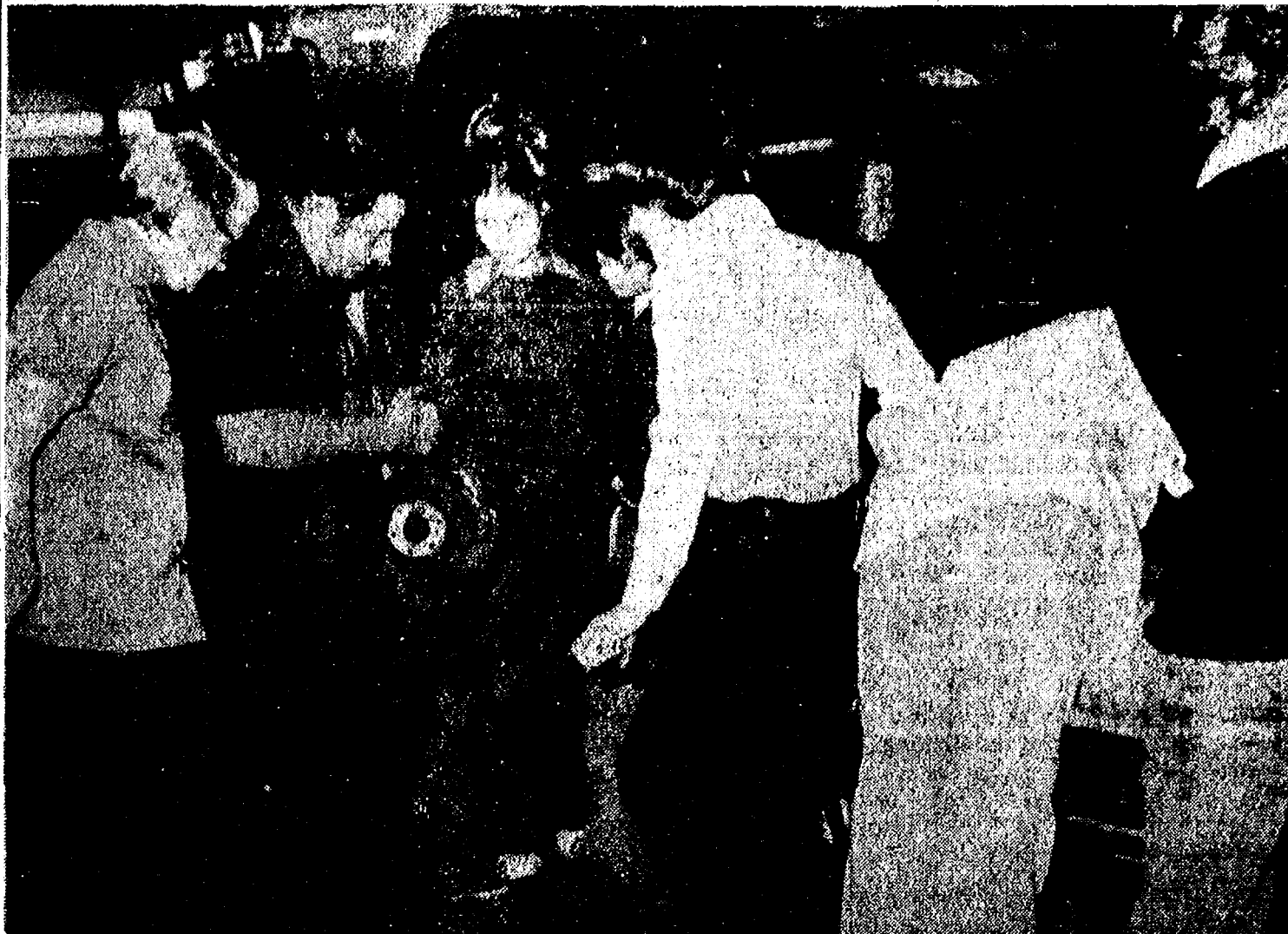
POWDER PUFF AUTO MECHANICS is the name given to the Chelsea Recreation Council course designed to familiarize women with their automobiles. Here instructor Bud Janich shows members of his class the fly wheel to which the starter is attached. Janich explains what actually happens when they put the key in the ignition, turn it, and start the car. Pictured from left, Millie McFadden, Janich, Stephanie Aldrich, Judy Staebler, Kathy Frisinger, Karen Kern and Sue Wood. There are 13 women now enrolled in the course.
